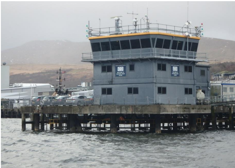
Figure 2 – QHM Clyde Port Operations – HMNB Clyde
